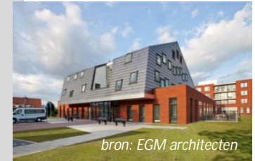
zorgcomplex Ameide Open Vensters bron: EGM architecten
